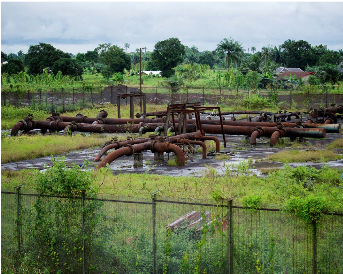
Shell's pipelines in Ogoniland are old and poorly maintained. There have been several spills and in 2009 there was a huge fire, at the Bomu Manifold, at K. Dere, Rivers state. September 2015. © Michael Uwemedimo/cmapping.net
